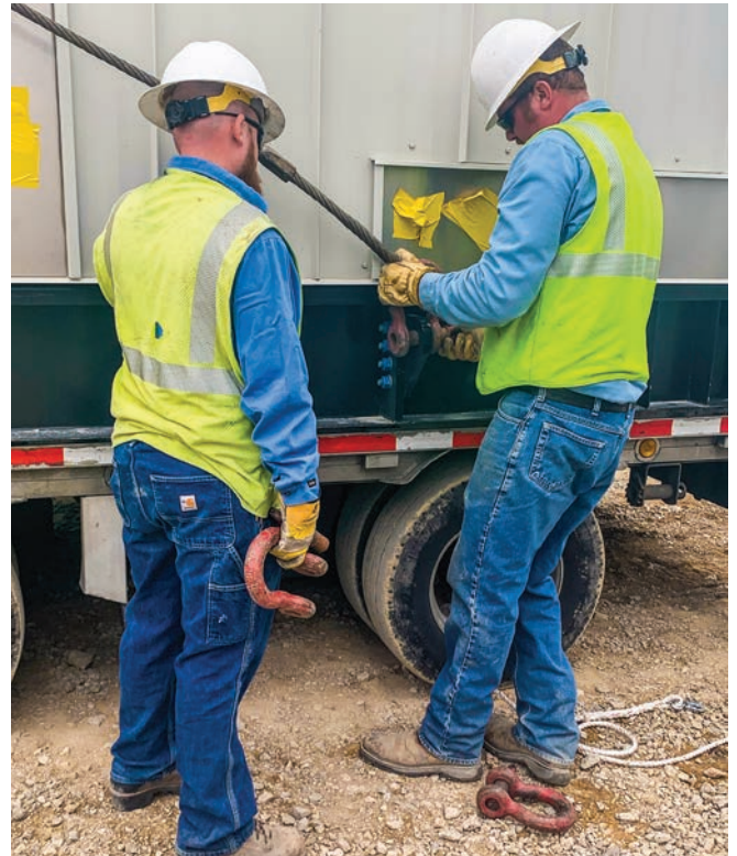
Journeyman linemen work to safely secure hooks prior to the crane (pictured below) lifting the generator from the special delivery trailer onto the concrete pad at the substation.
