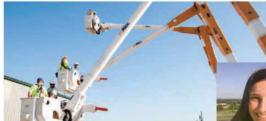
FreeState Electric linemen give safety demonstrations and bucket truck rides to teach the 40 Kansas/Hawaii Youth Tour delegates about electric co-ops.
